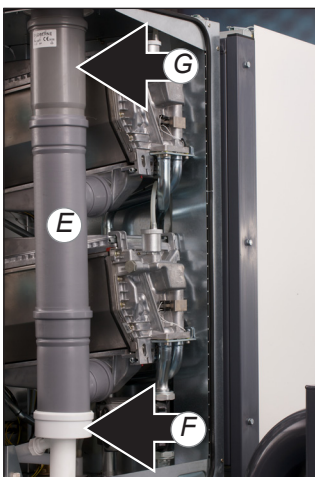
Removing flue pipe
